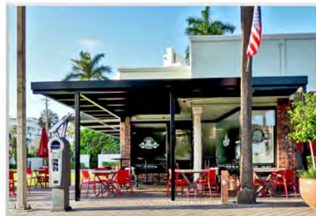
METAL ROOF & CANOPY FORT LAUDERDALE, FLORIDA
